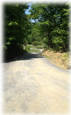
Below Photograph: Shows re-graded Spring Park Trail and newly dug ditch line to protect new line.
